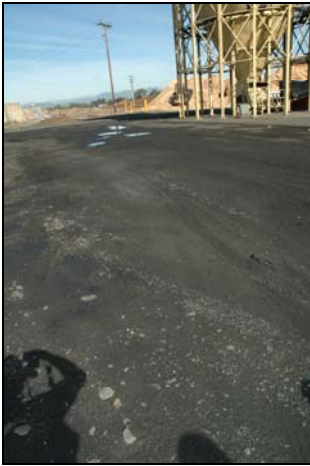
Photo 2: Organic ash located on the surface of the subject property viewing in a northerly direction.
