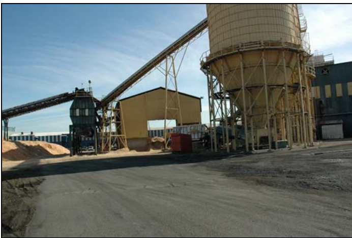
Photo 3: Roadway and operations adjacent north of the subject property.
