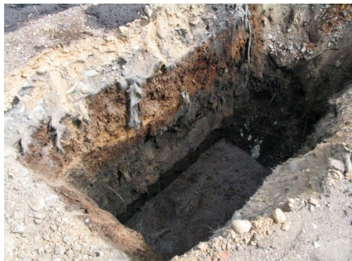
Figure 1: Profile of test hole 1, facing NE corner (piling removed)
