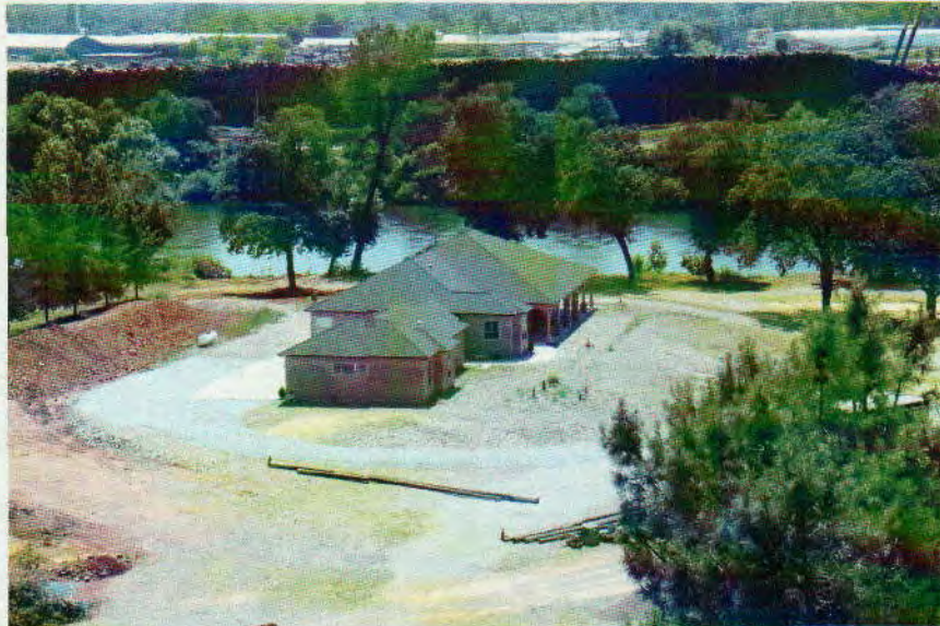
JGW RV Owner Residence- see SP LOG PILES across river
