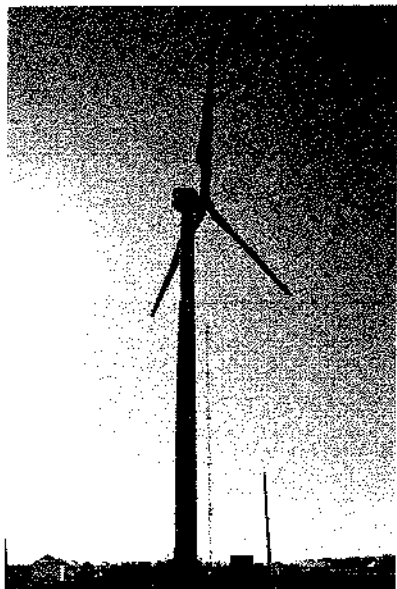
Utility-Scale Wind turbine with an anemometer tower in the background. Credit: University of Minnesota College of Science and Engineering
