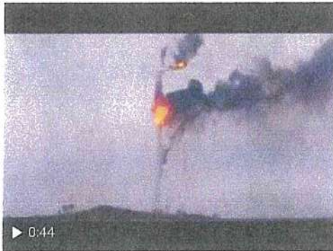
WindTurbine on fire - YouTube The Weather Channel
