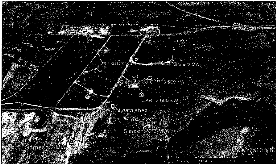
FIGURE 1 National Wind Technology Center (NWTC) row 4 wind turbines [Colour figure can be viewed at wileyonlinelibrary.com]
